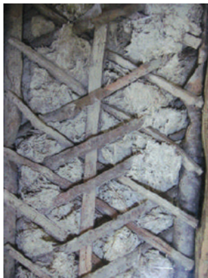
Figura 3.5 - parede wattle and daub.
