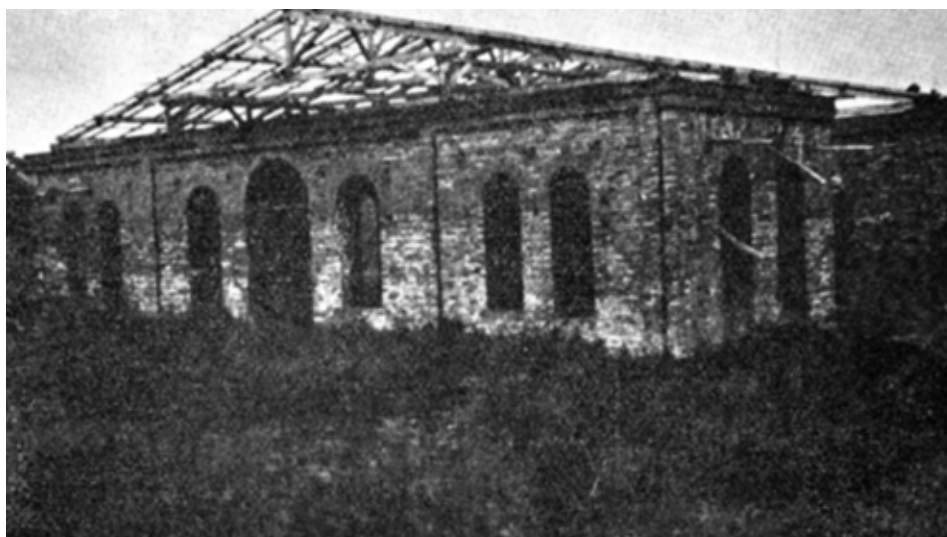
Fig.55 – Customs (abandoned before finished).
