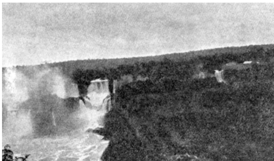
Fig.62 – Iguazu Falls, hotel, and police station in Argentina.
